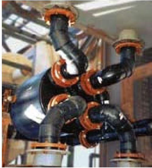
Prefab Piping Spools
