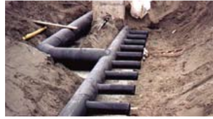
Odor Control (Foul Air) / Biofilter Systems
