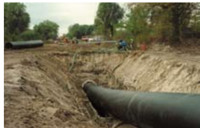
Sanitary Sewer & Insert Renewal
