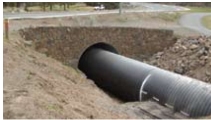
New Culvert & Culvert Relining
